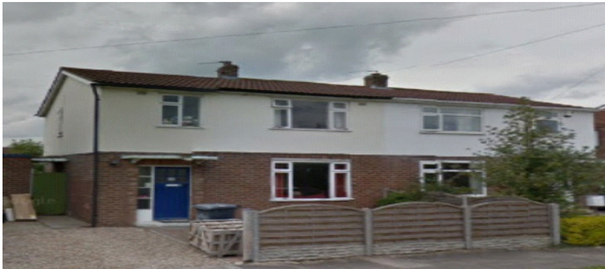
Figure 5 – Showing a spooner type property on Leven Road
