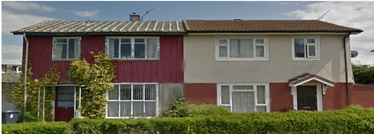
Figure 1 - An example of a BISF house on Danebury drive
